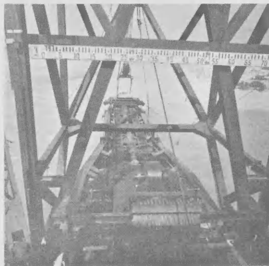
This is the 84-foot shaft with cutter of dredge "Georgia" with depth scale.
